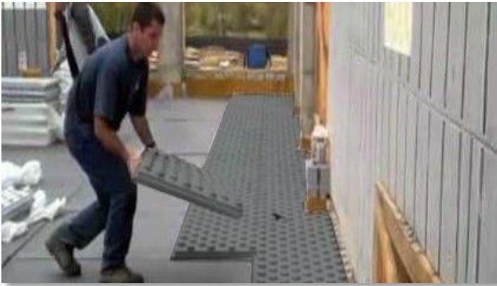
Radiant Floor Panels
