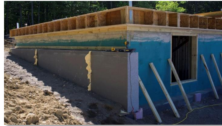
Exterior Basement Wall
