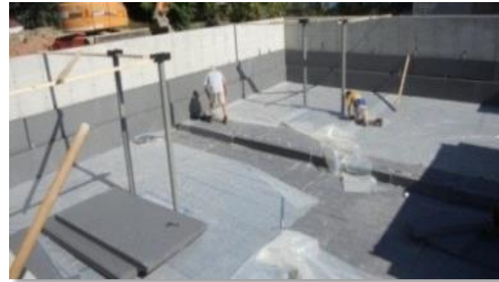
Interior Basement Wall
