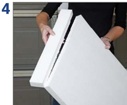
Break off the insulation where cut.
