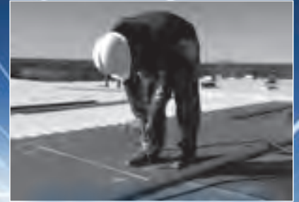
Roofing - New and Retrofit
