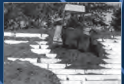
Geofoam - Lightweight Void Fill
