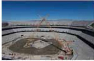
Football Stadium, CA
